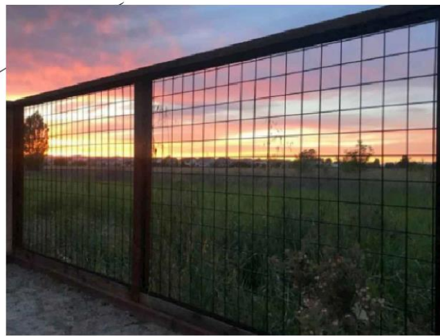
HOG WIRE FENCING WITHIN METAL FRAMED PANELS
