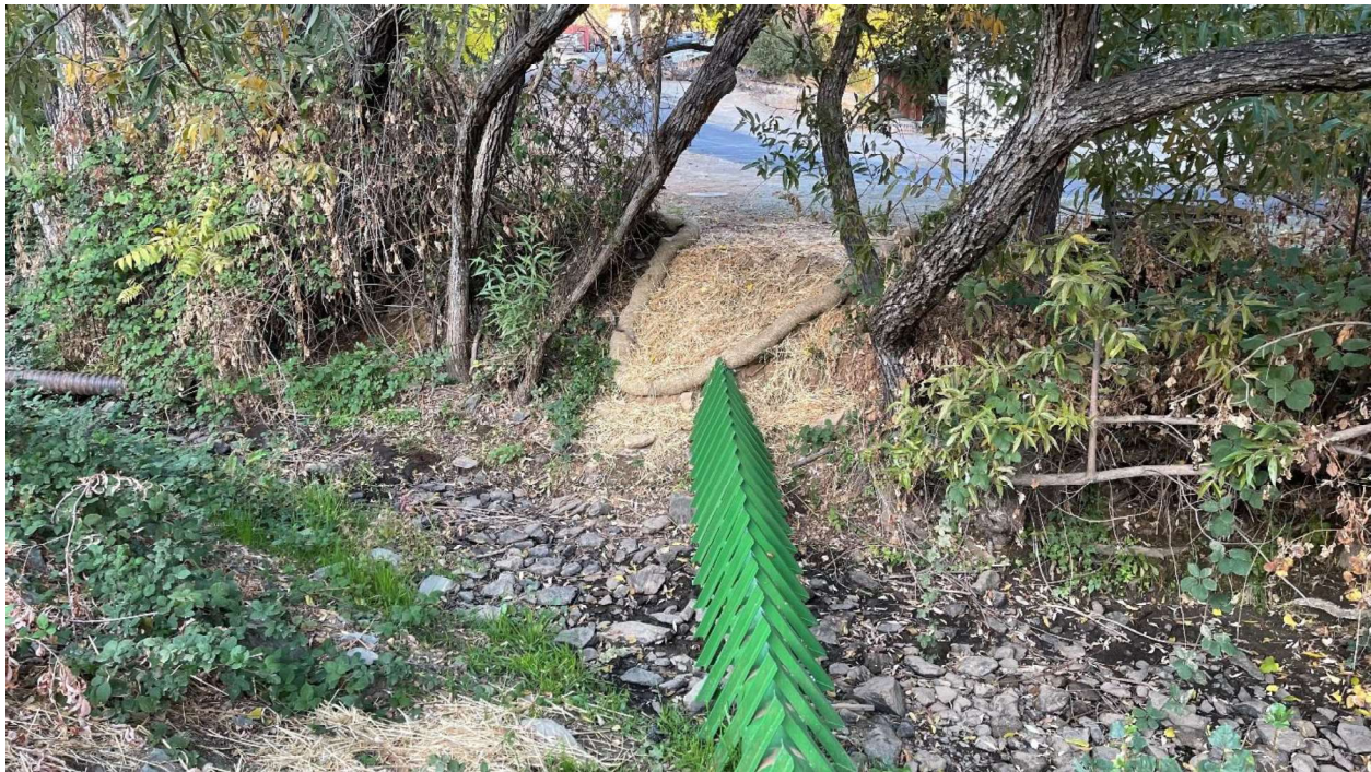
11. Slope erosion control at China Gulch Sewer Crossing
