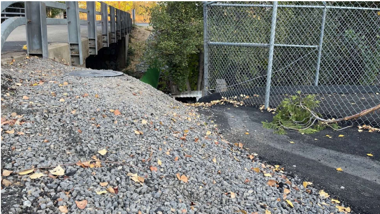
10. AC paving and rock placed to protect bank of Angels Creek
