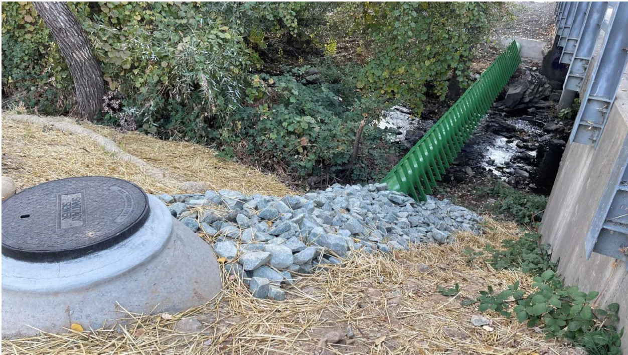
7. Rock slope protection provided along bank of Angels Creek
