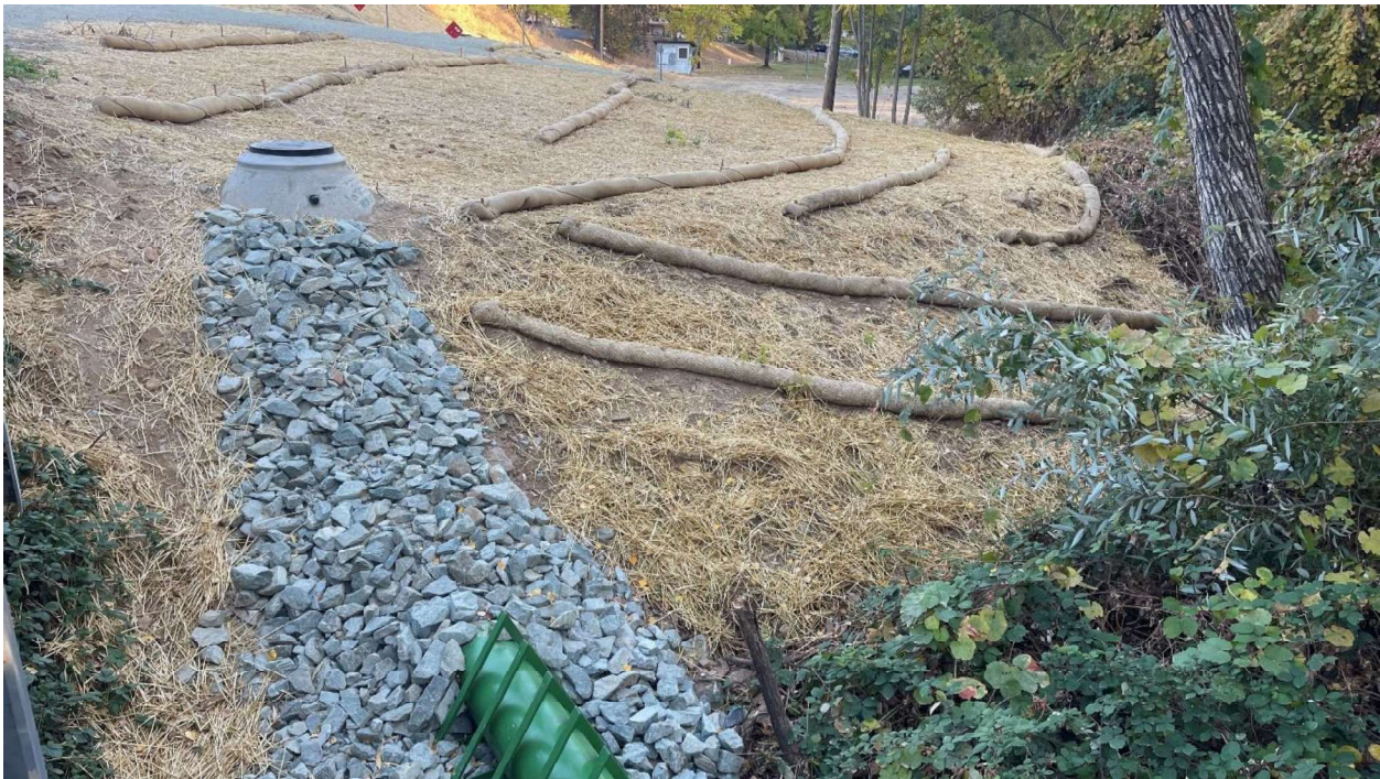
8. Rock slope protection provided along bank of Angels Creek
