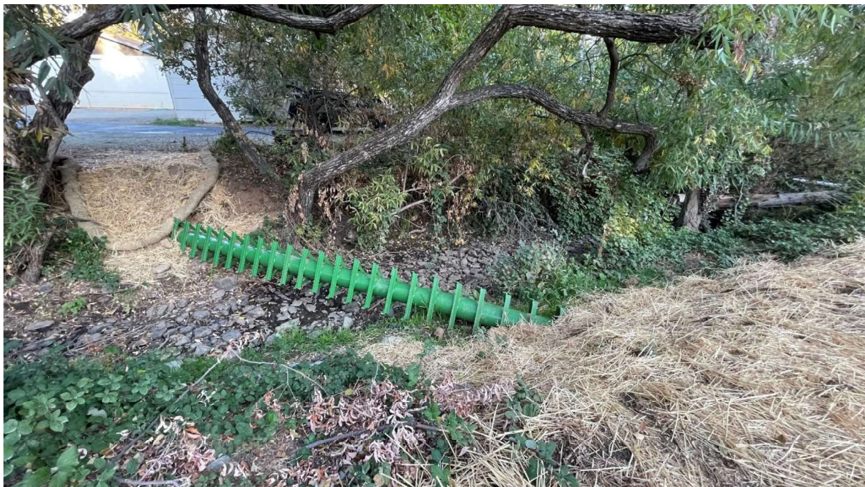
12. Slope erosion control at China Gulch Sewer Crossing
