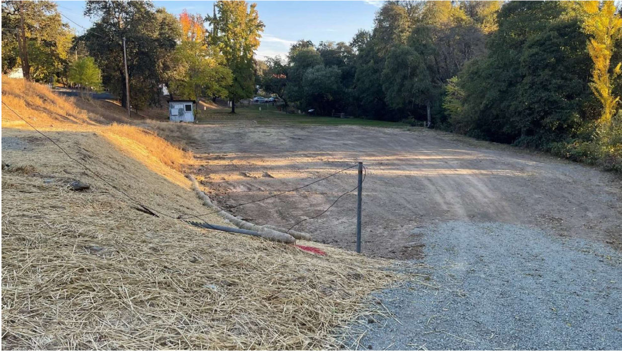
1. Erosion control and all-weather road at park entrance
