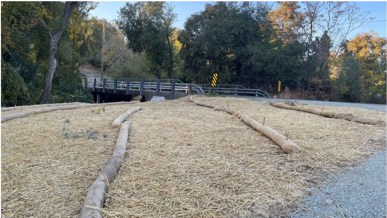
6. Erosion protection provided to facilitate access to manhole
