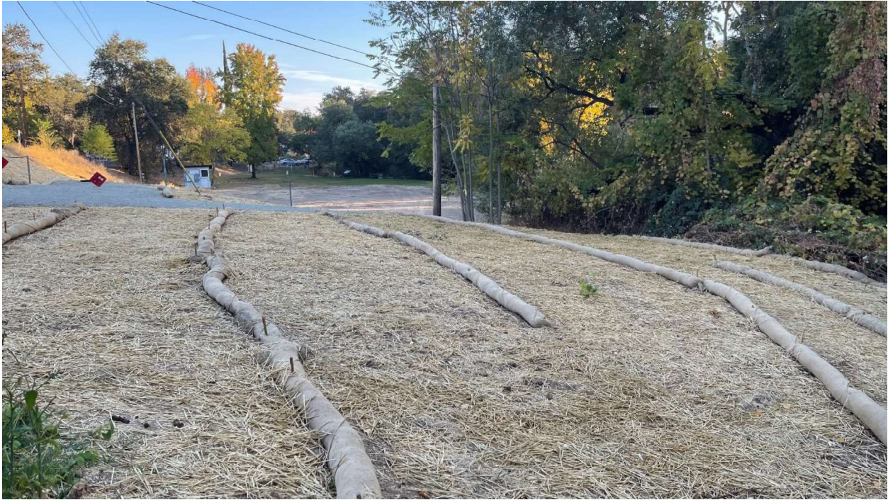
5. Erosion protection provided along bank of Angels Creek
