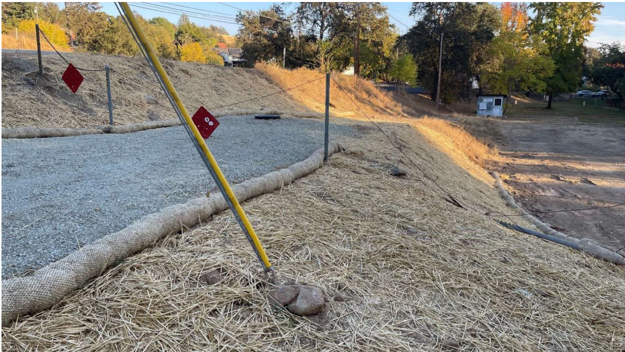
2. Erosion control and all-weather road materials constructed to facilitate access to manhole
