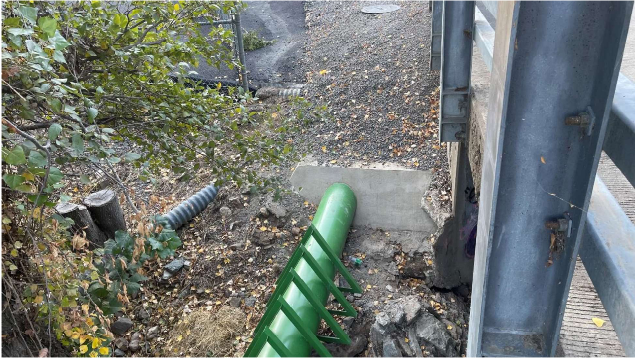
9. Concrete headwall constructed to protect pipe/bank at Angels Creek
