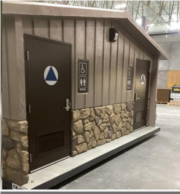
Figure 2: Utica Park New Bathroom (Actual, Constructed)
