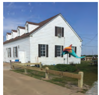
Light wood guardrail at Little Island Park
