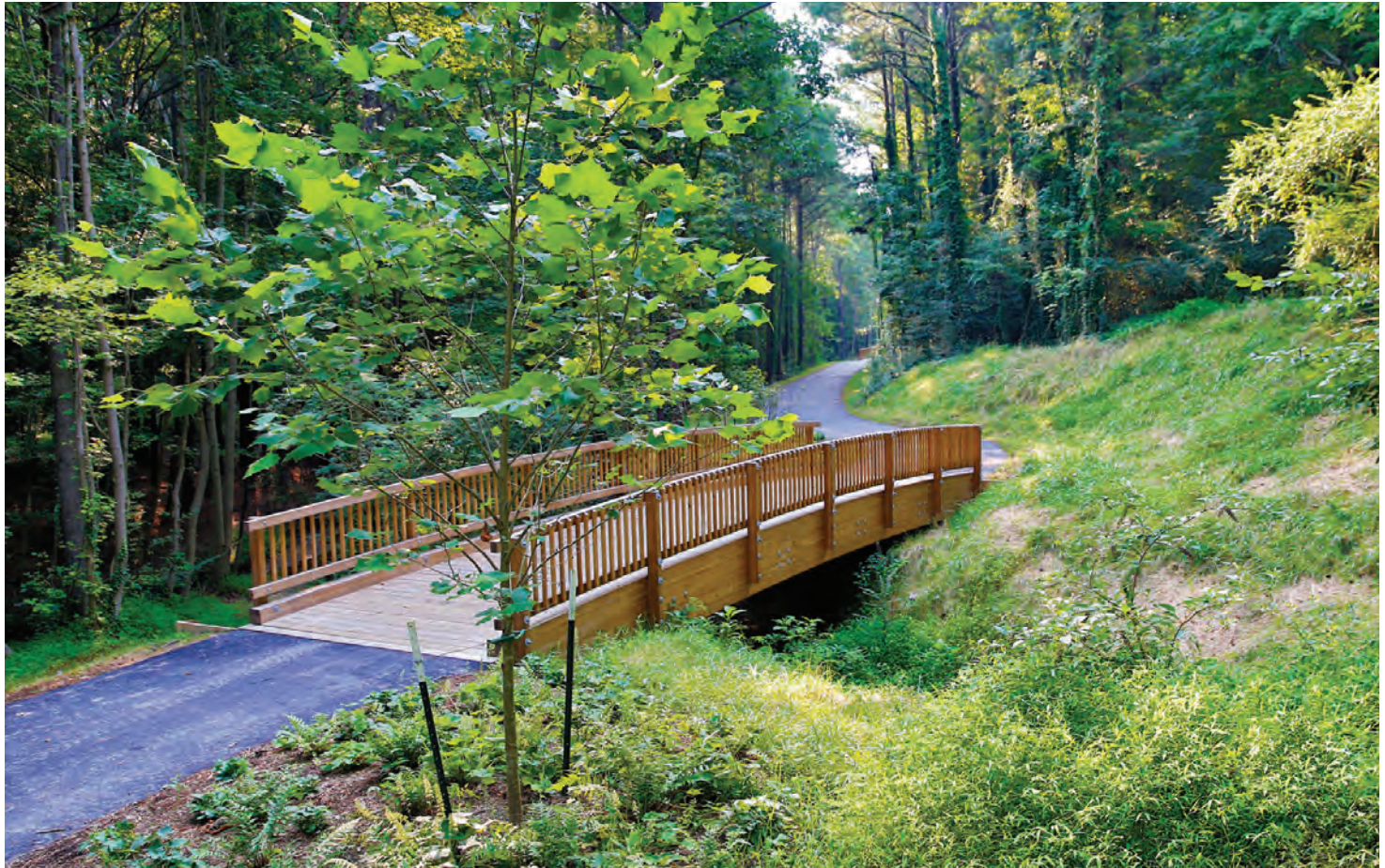
Prefabricated bridge at Marshview Park
