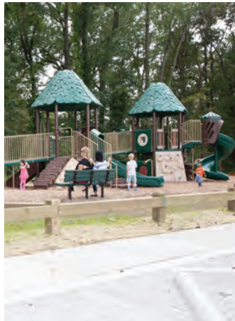
Typical wood guardrail at Lake Lawson/Lake Smith Natural Area playground
