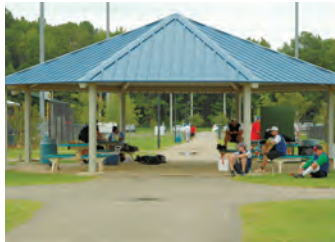
Metal shelter at Princess Anne Athletic Complex
