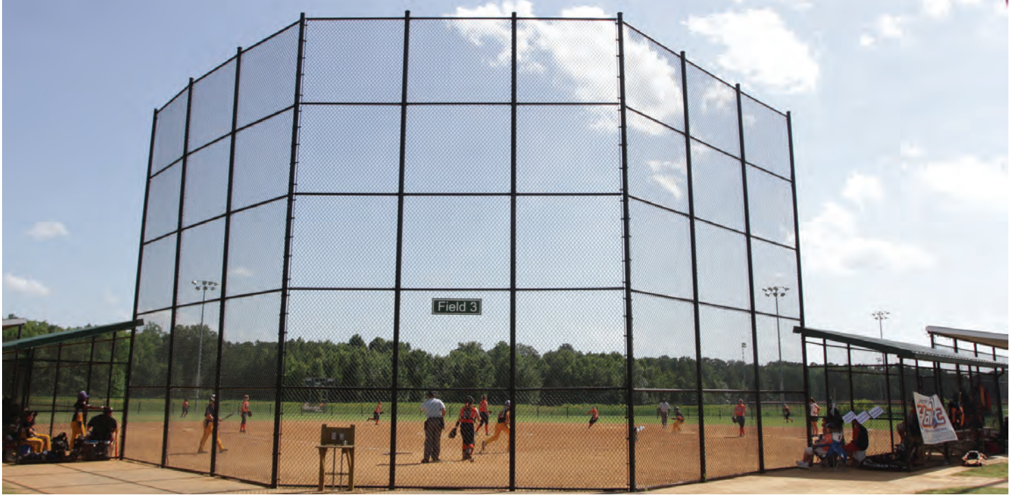
(Top photo): Extended backstop at Princess Anne Athletic Complex
