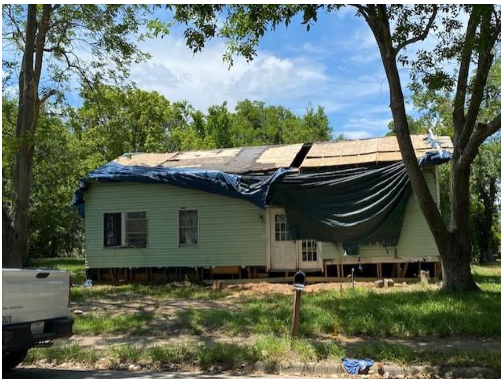
Roof missing and plywood separated, continued exposure of interior of structure to external elements
