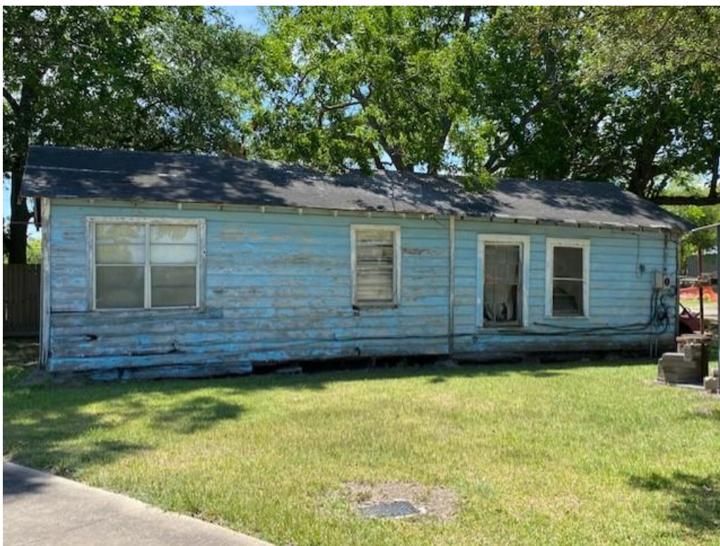
Back side of house – extensive wood rot, holes in roof, missing windows, floor and siding deterioration
