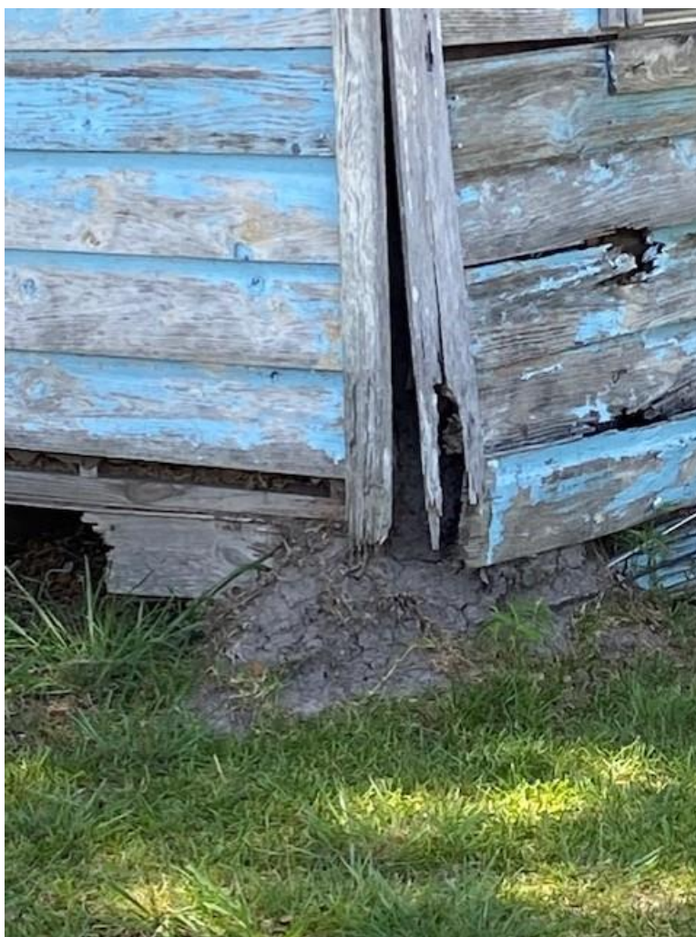
Insect mound, separated corner, rotted floor and beams, wood rot
