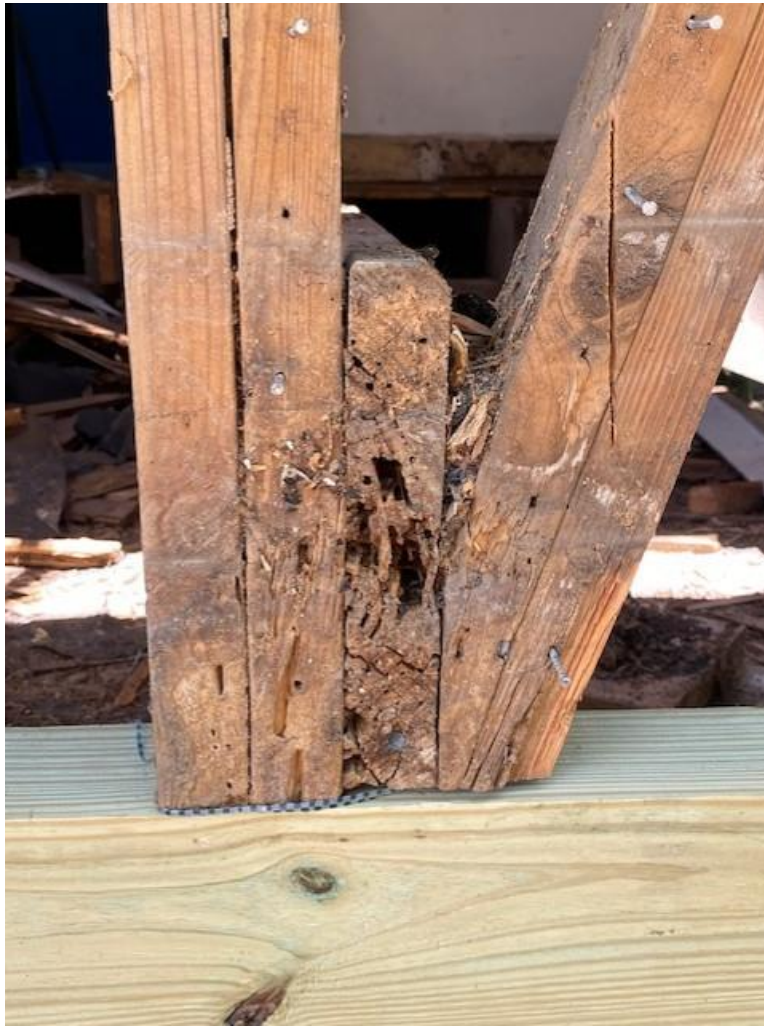
Termite damage - structural beam
