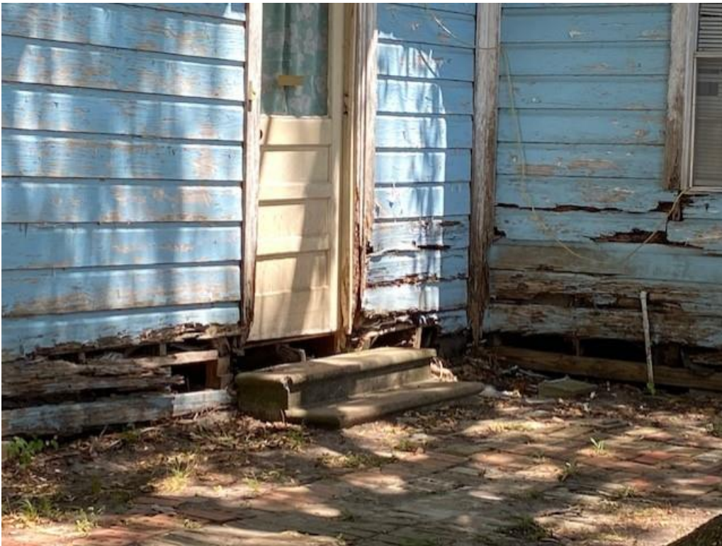
Front close-up – extensive wood rot
