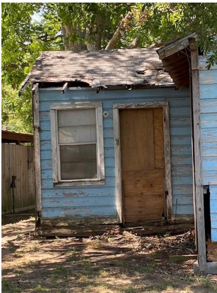
Back door missing, holes in roof, rotted/missing eaves, wood rotted siding
