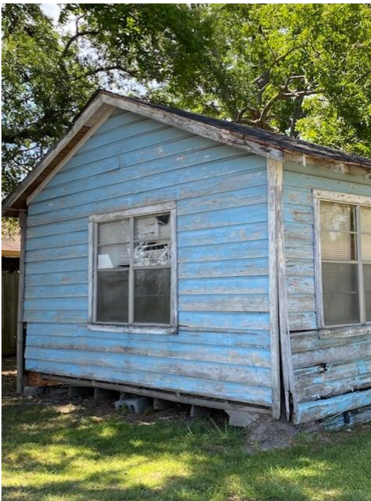
South side of structure, separated corners filled by insect mound, missing windows, rotted roof eaves.
