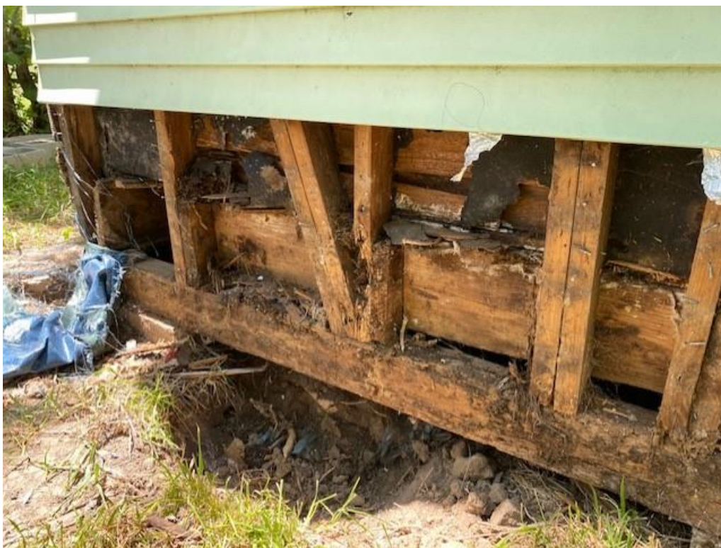
Structural wood rot and missing siding
