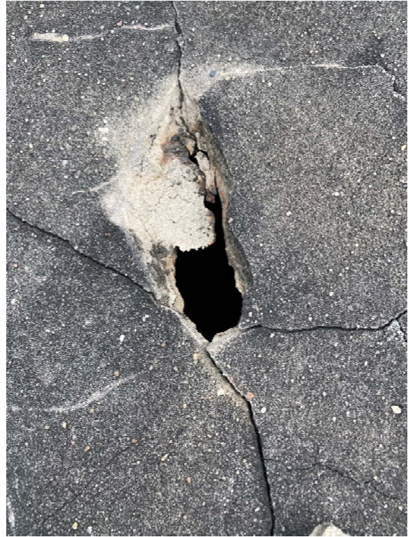
Close up of Cracking and Loose Gunite on the Dome from Photo Above
