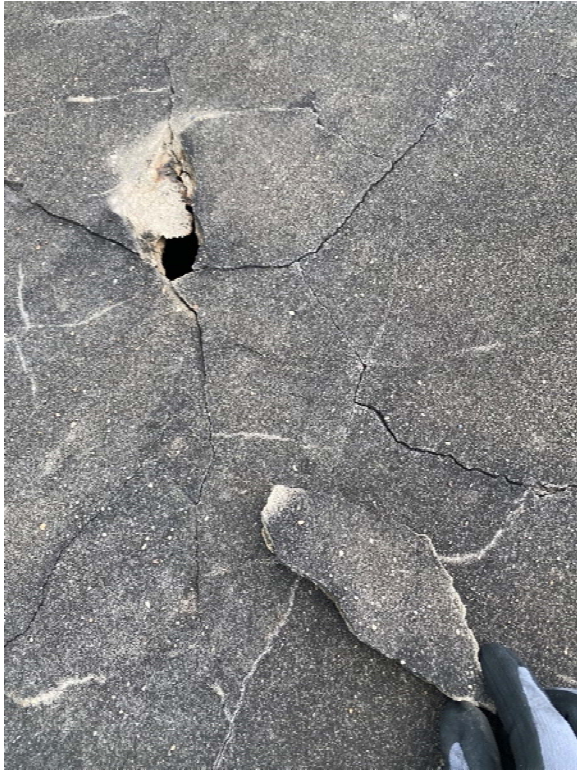
Close up of Cracking and Loose Gunite on the Dome from Photo Above
