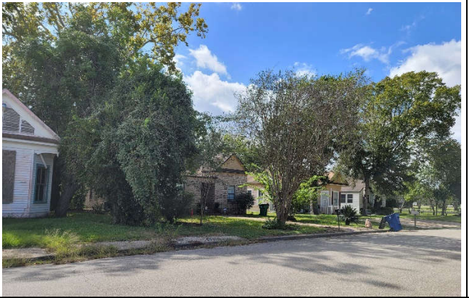
VIEW LOOKING SOUTHWEST @HOMES NEXT DOOR
