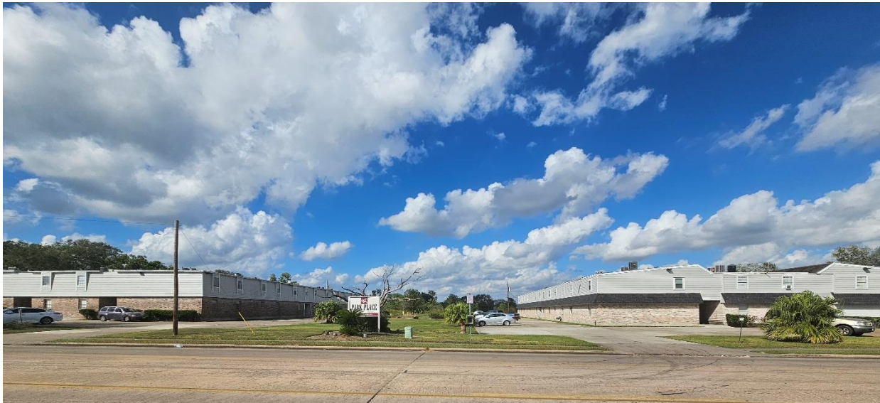
View looking north from Cemetery Rd. from property frontage
