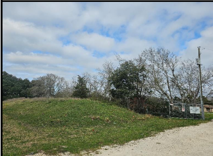
View looking East from Site @ Berm area
