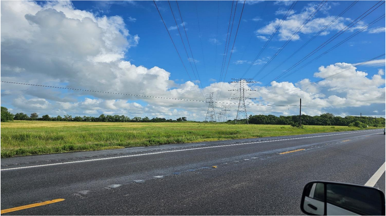
View looking northwest toward Site from SH 35
