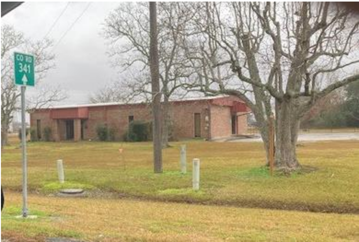
View of Site from SH 35
