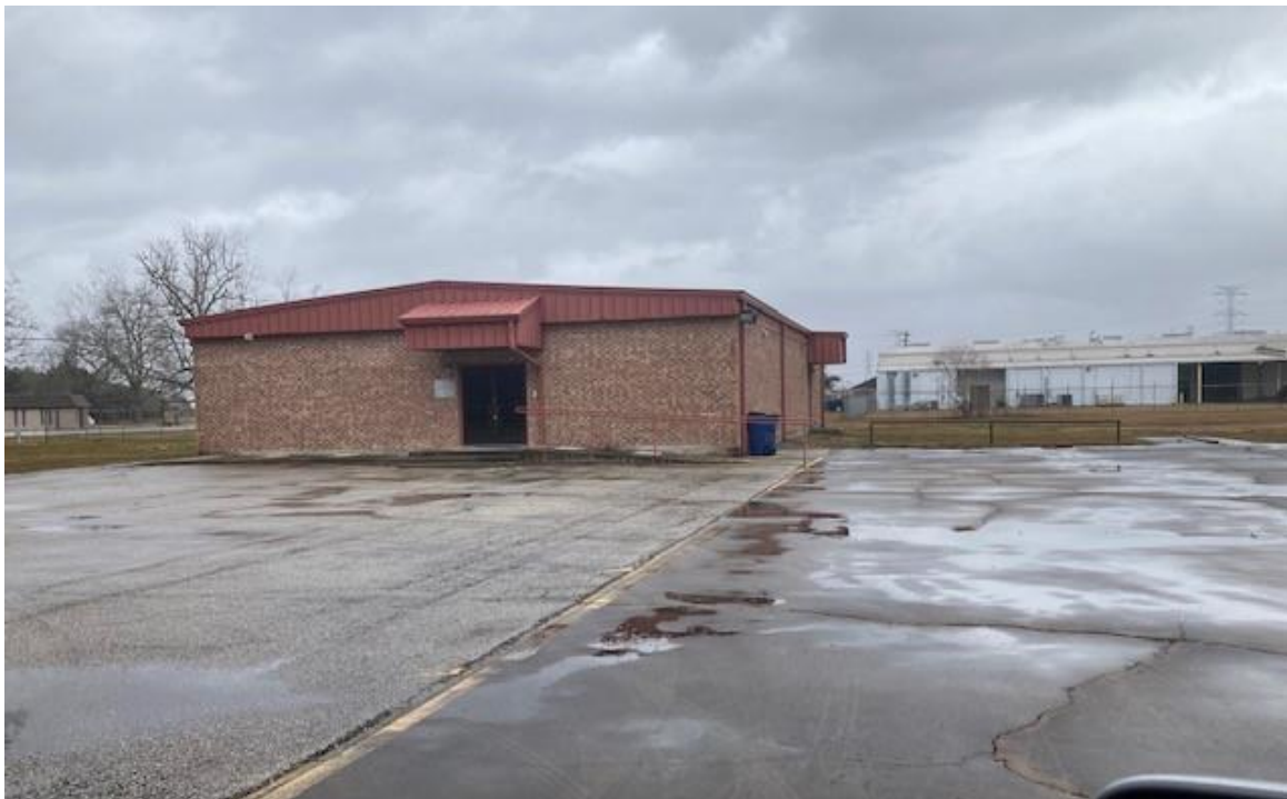
View of building and parking lot from Rab Rd.
