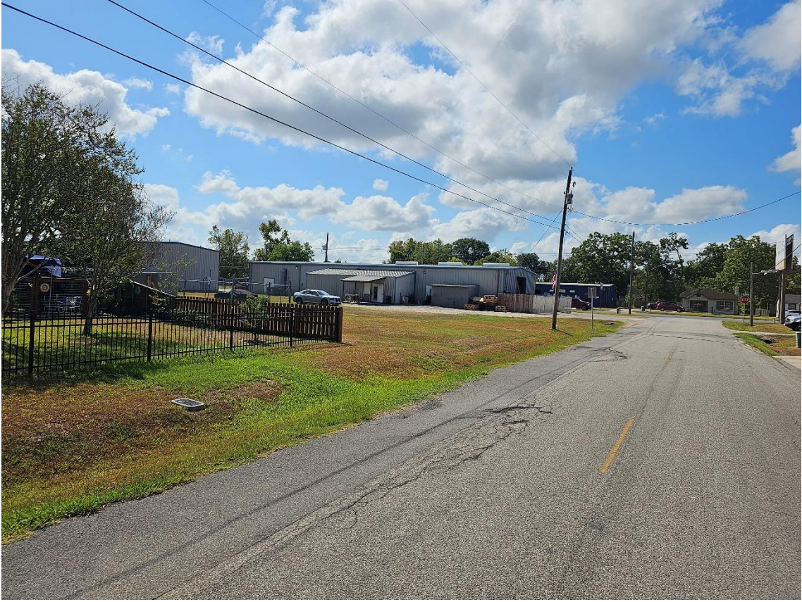
View facing South, showing behind business
