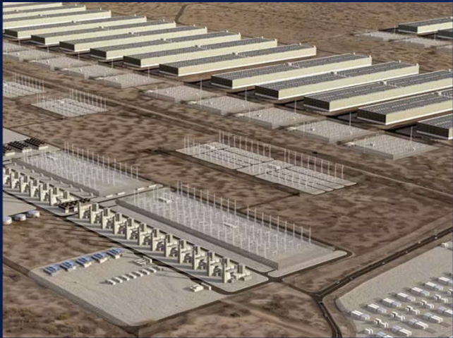
The GW Ranch (a private-grid power generation campus under development by Pacifco Energy in Pecos County, Texas).
