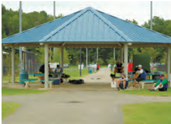
Metal shelter at Princess Anne Athletic Complex
