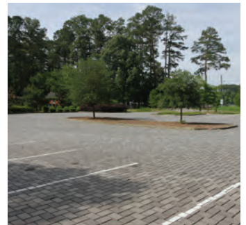
Pervious parking lot at Stumpy Lake Natural Area
