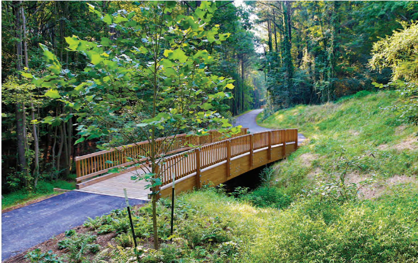
Prefabricated bridge at Marshview Park
