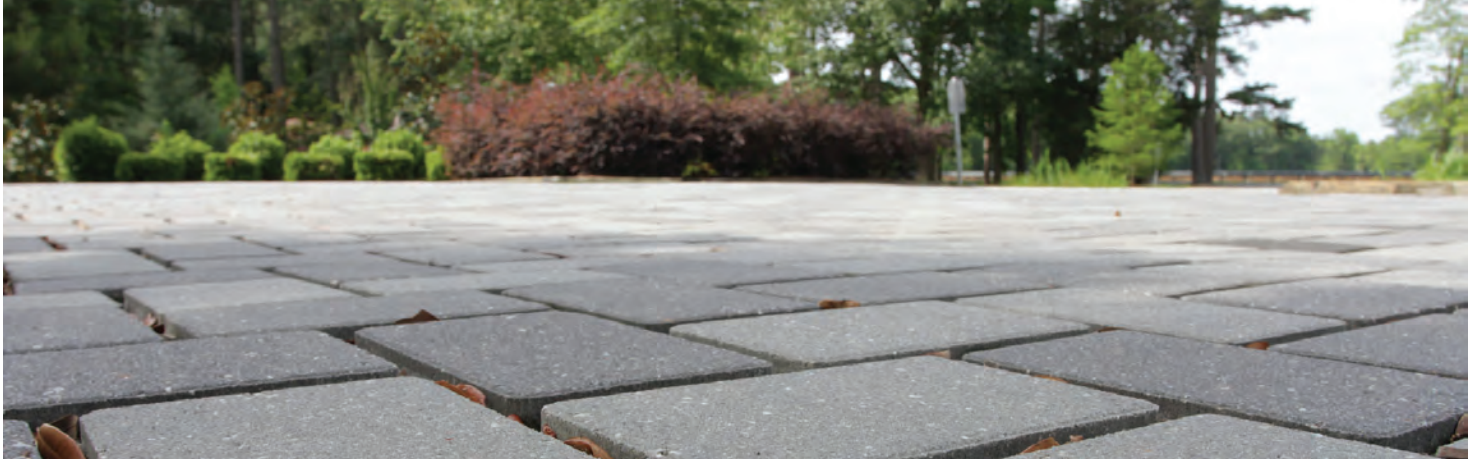
Pervious parking lot at Stumpy Lake Natural Area
