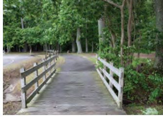
Foot Bridge at Red Wing Park
