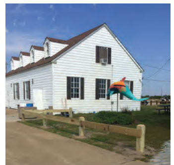
Light wood guardrail at Little Island Park
