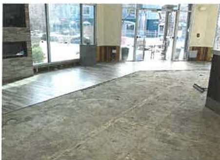
Lobby; first responder equipment removal
