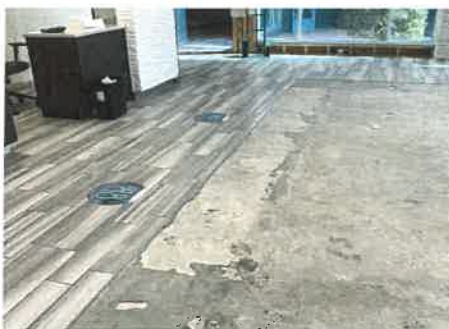
Lobby; first responder equipment removal
