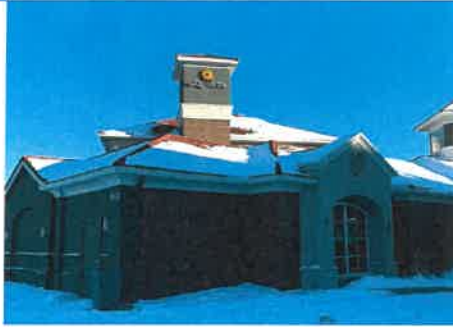
Front of structure
