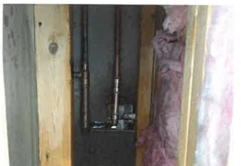
Lobby; plumbing repair
