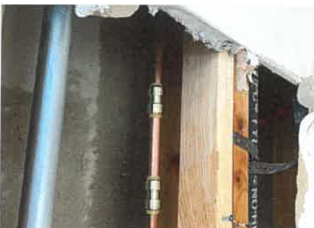
Lobby; plumbing repair
