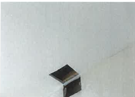
Lobby; plumbers cuts
