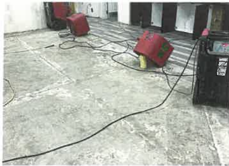
Lobby; first responders equipment
