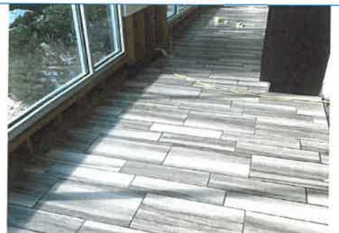
Lobby; first responder equipment removal
