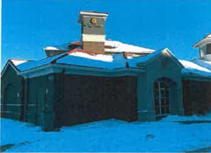
Front of structure
