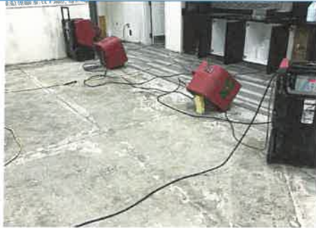
Lobby; first responders equipment
