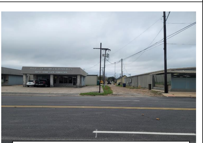
VIEW LOOKING WEST TOWARD SITE
