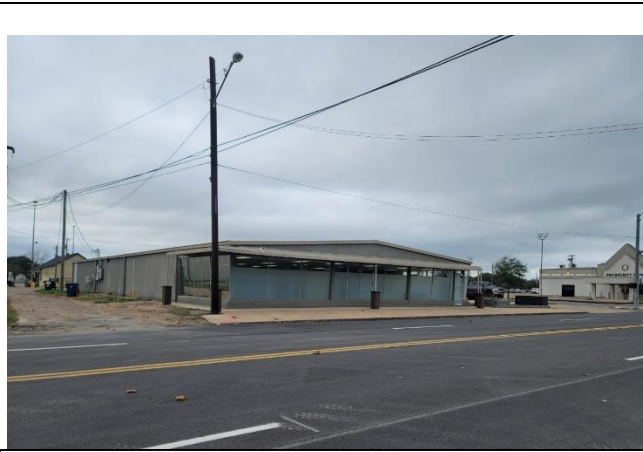
VIEW LOOKING WEST @ SITE
