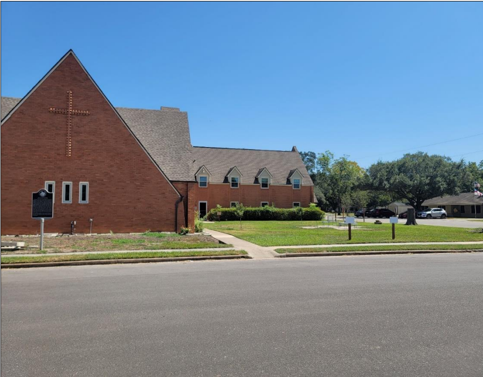
View from S. Chenango St. looking towards the Church
