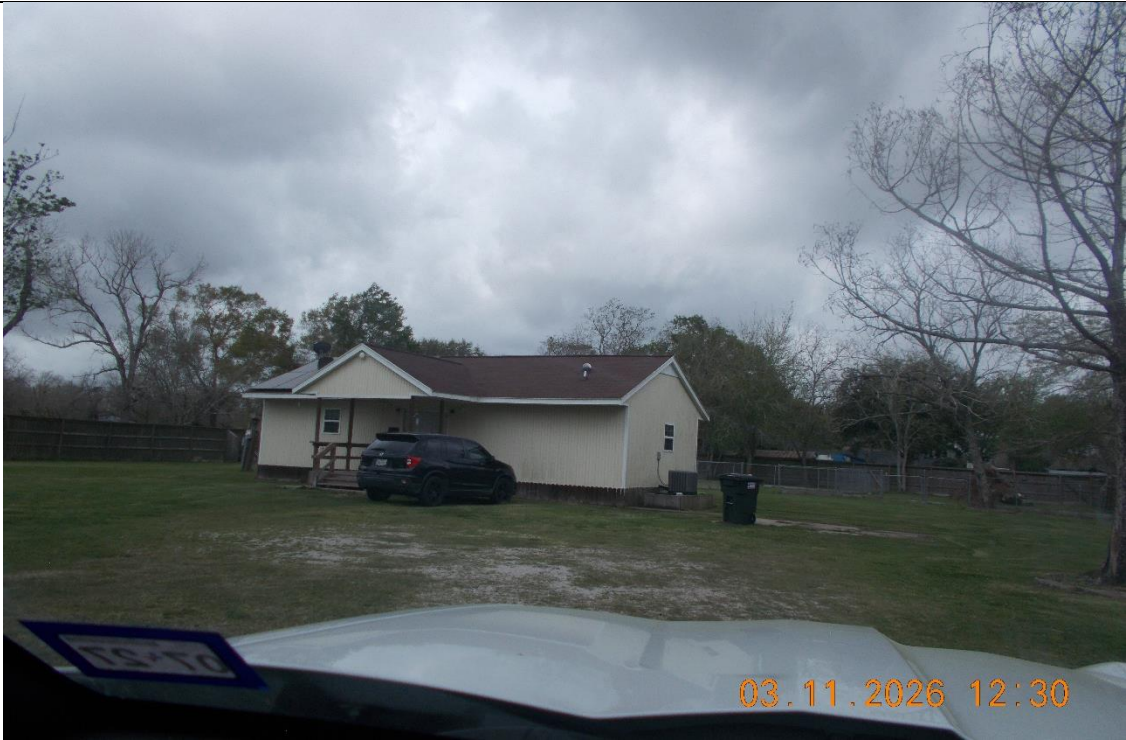
View of site looking at rear home structure
