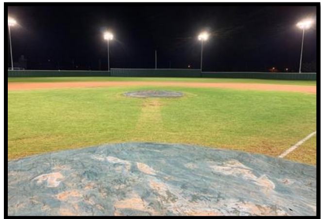
Pearsall ISD Sports Lighting Upgrade Project
