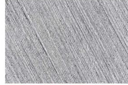
BROOM FINISHED CONCRETE PAVING
