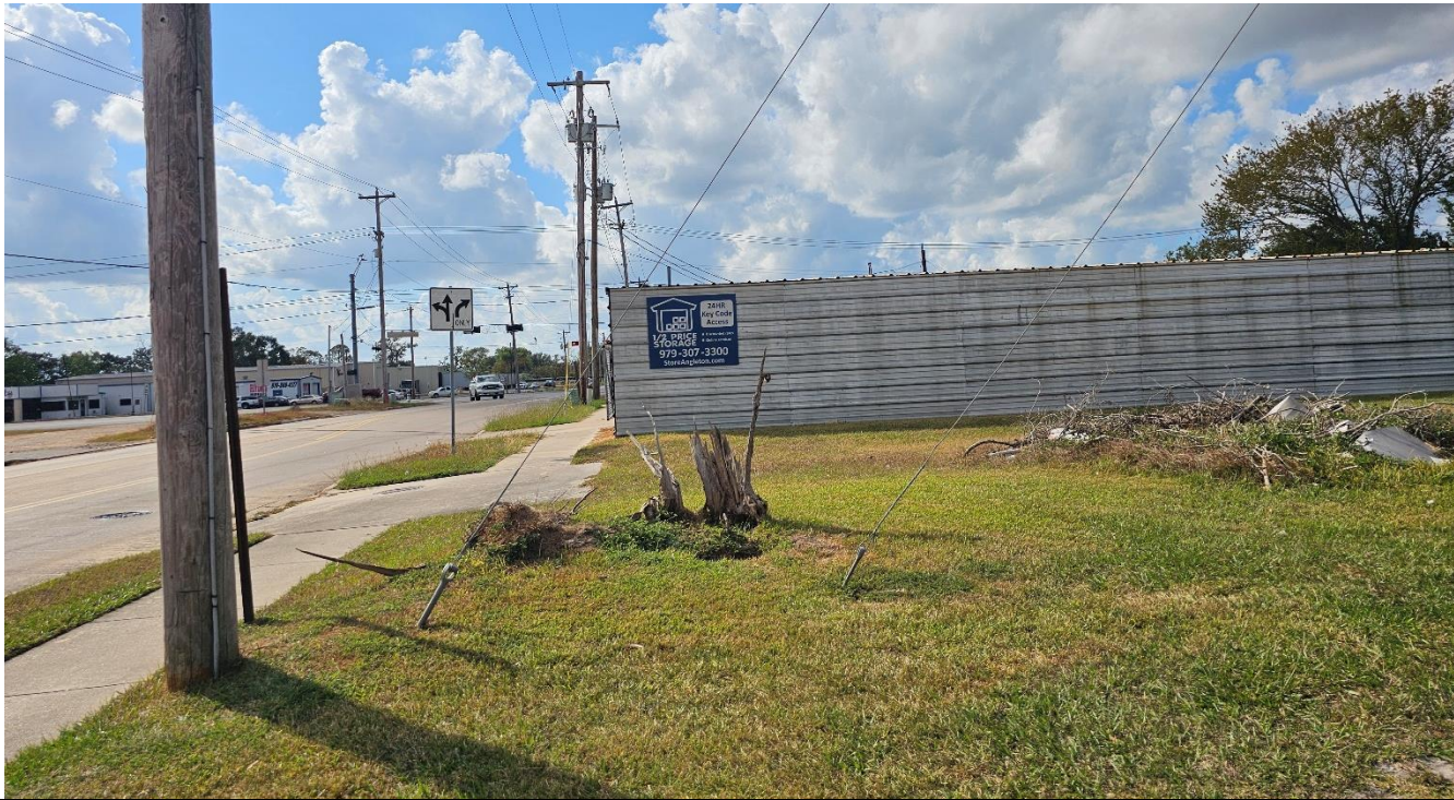
View looking West on Cemetery Rd. toward SH288 B, Mini-Storage Units to the right
