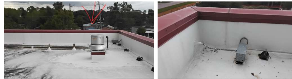
Backside @ rooftop parapet wall - For Reference
