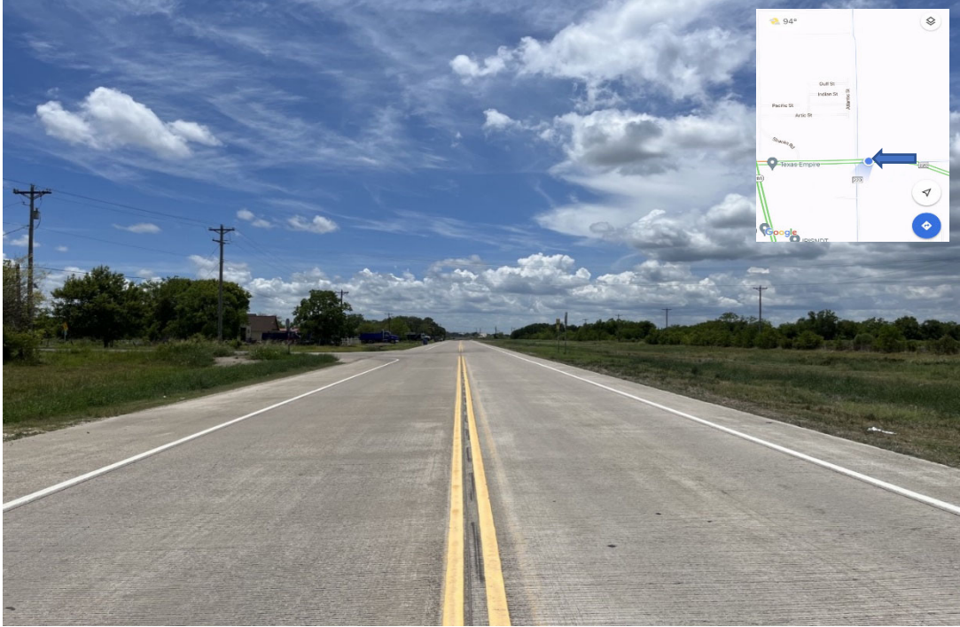
Figure A1. CR220/Coale Rd. Westbound Approach
