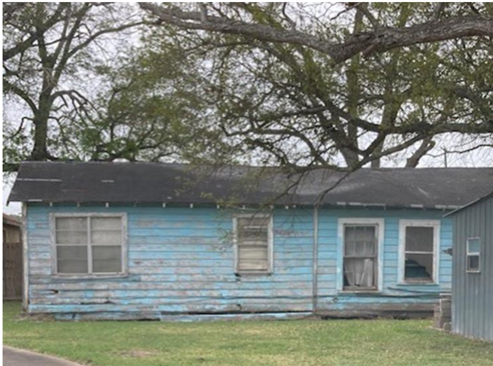
Siding rotted and holes in siding observed
