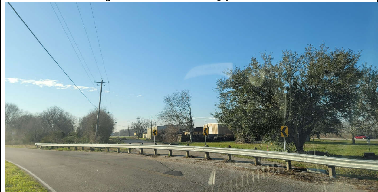
View looking south on Shanks Rd. @ point of road extension
