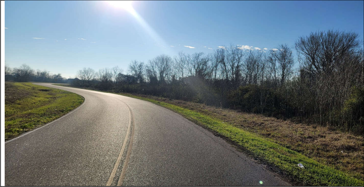
View looking south along the Shanks Rd. extension, Site on Right
