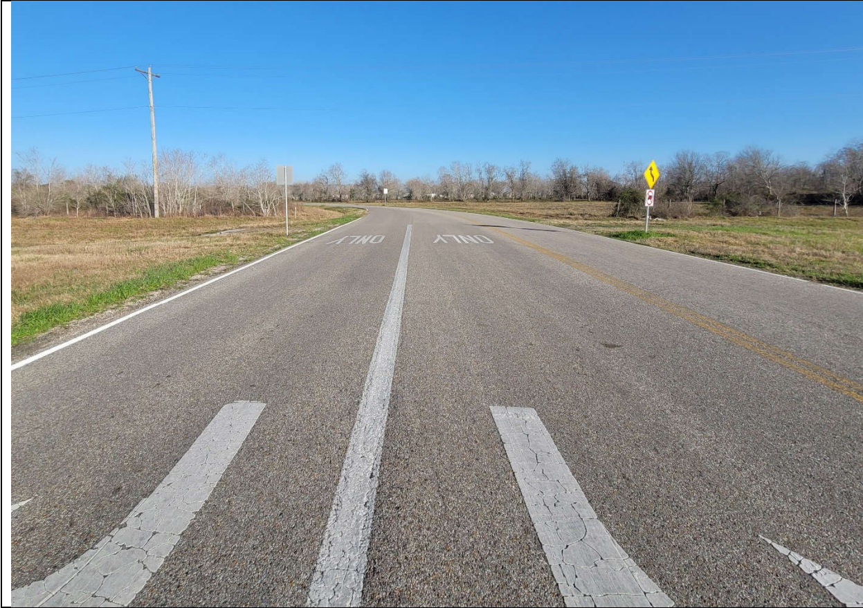
View looking north on Shanks Rd. at CR220, Site on left
