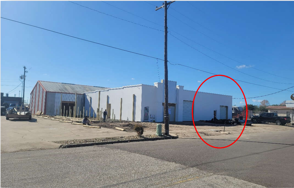
View of 117 West Myrtle Street, Looking at subject property, and site
