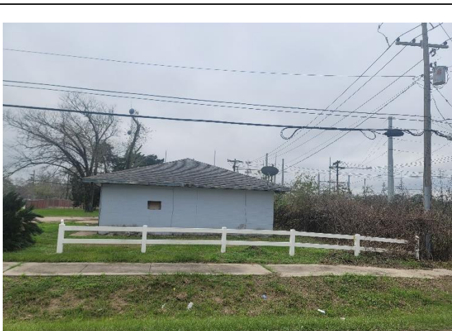
VIEW LOOKING SOUTH AT PROJECT SITE
