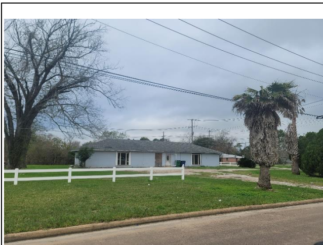
VIEW LOOKING WEST AT PROJECT SITE
