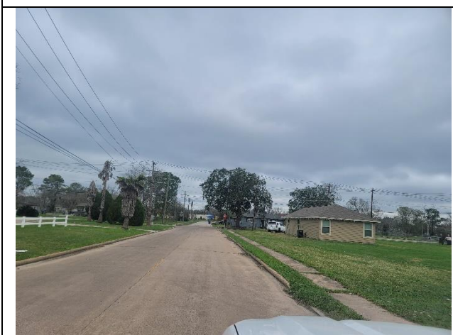
VIEW LOOKING NORTH ON WALKER ST.
