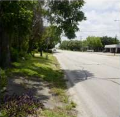
Existing Inconsistent Sidewalk
