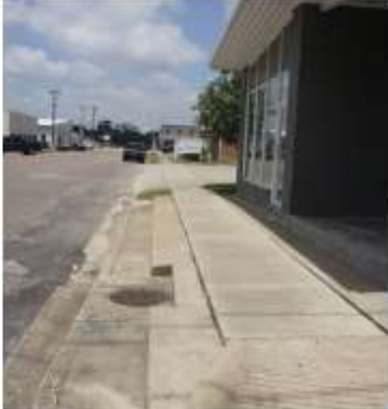
Existing High Sidewalk
