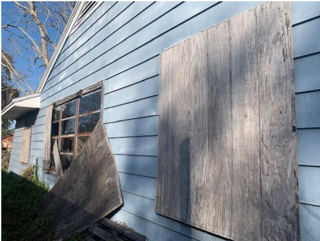
Windows boarded, windows broken, structure leaning
