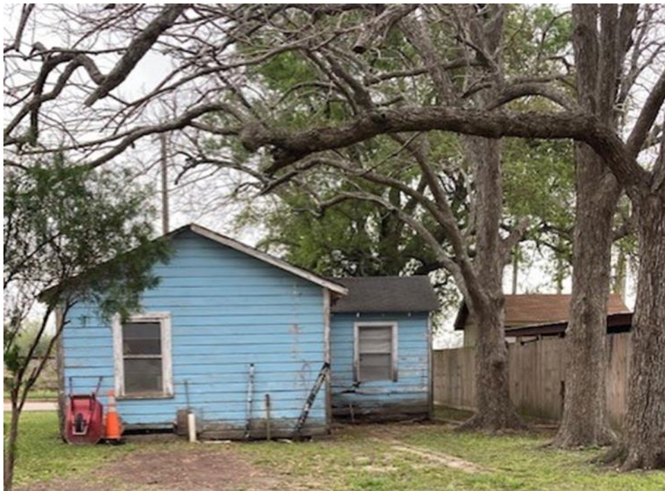
Rotted exterior siding, broken windows
