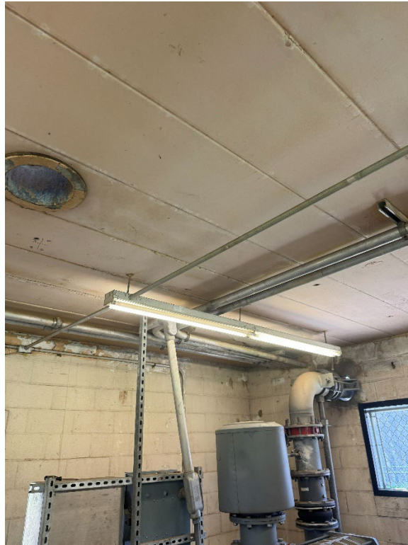
Figure 5 View of Blower Building ceiling and walls
