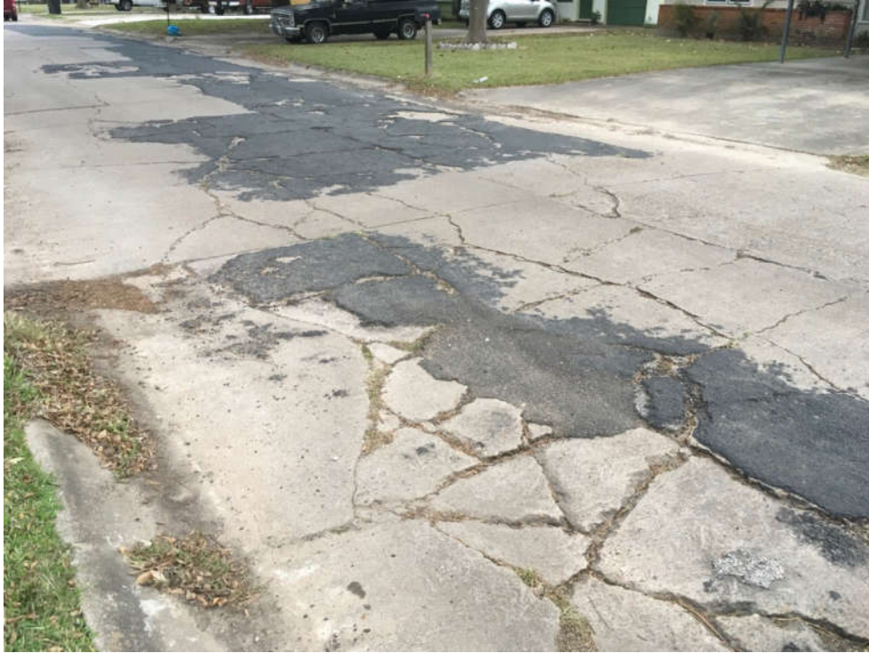
BLOCK CRACKING
