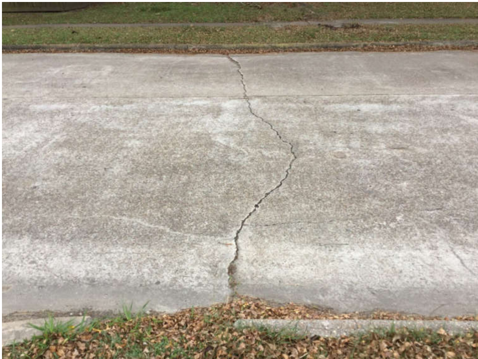
TRANSVERSE CRACKING
