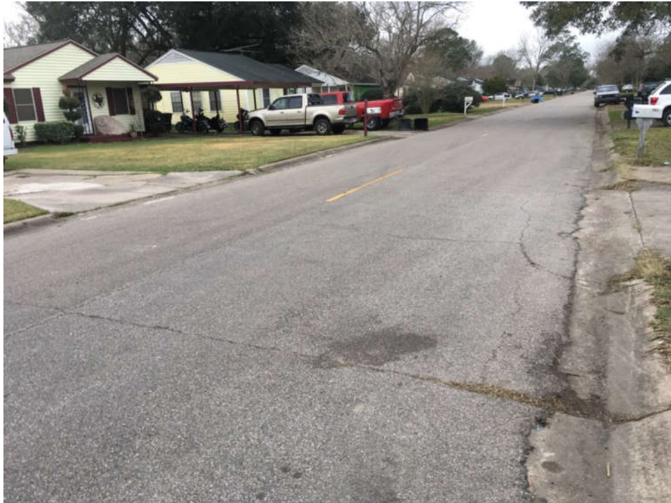
BLOCK CRACKING
