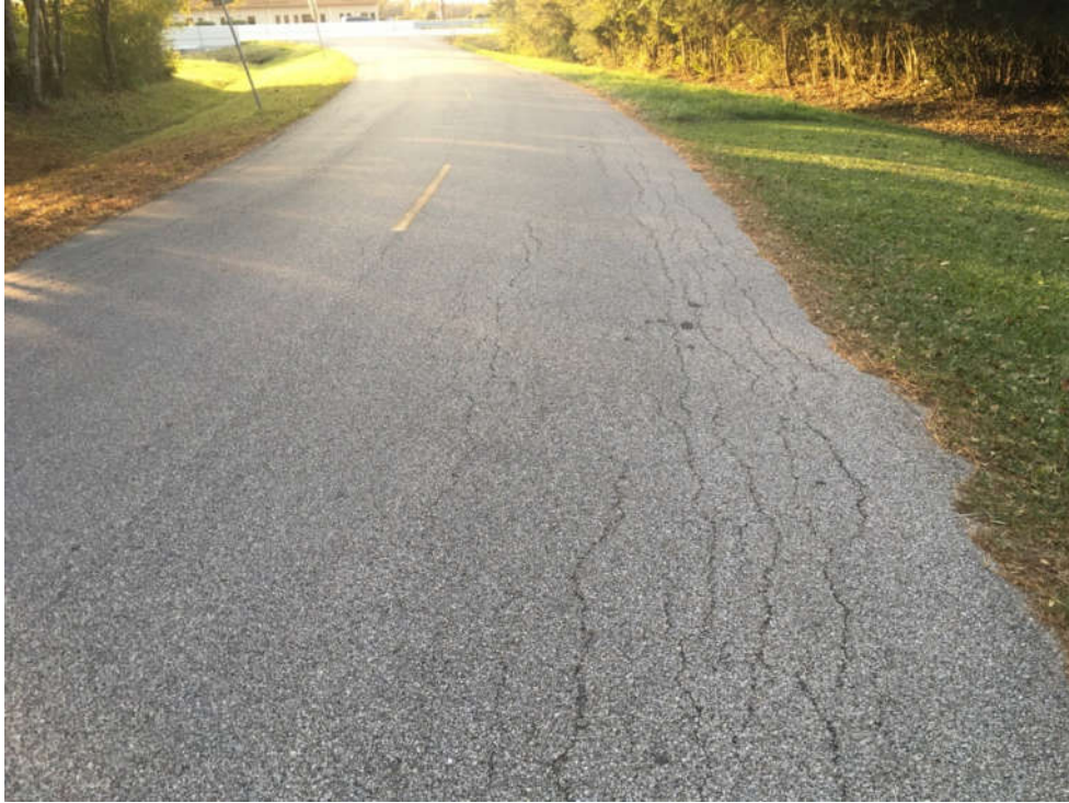
SLIPPAGE CRACKING
