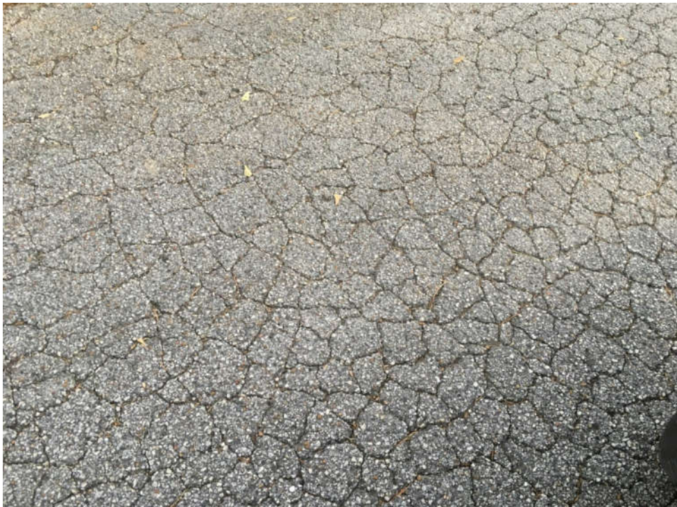
ALLIGATOR CRACKING
