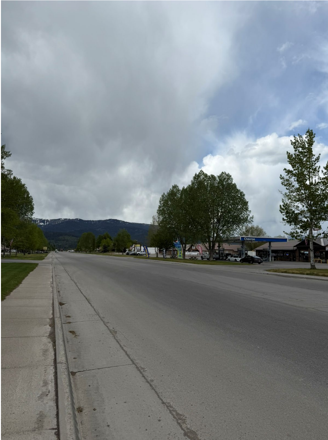
Figure 3. US 89 south of Center Street
