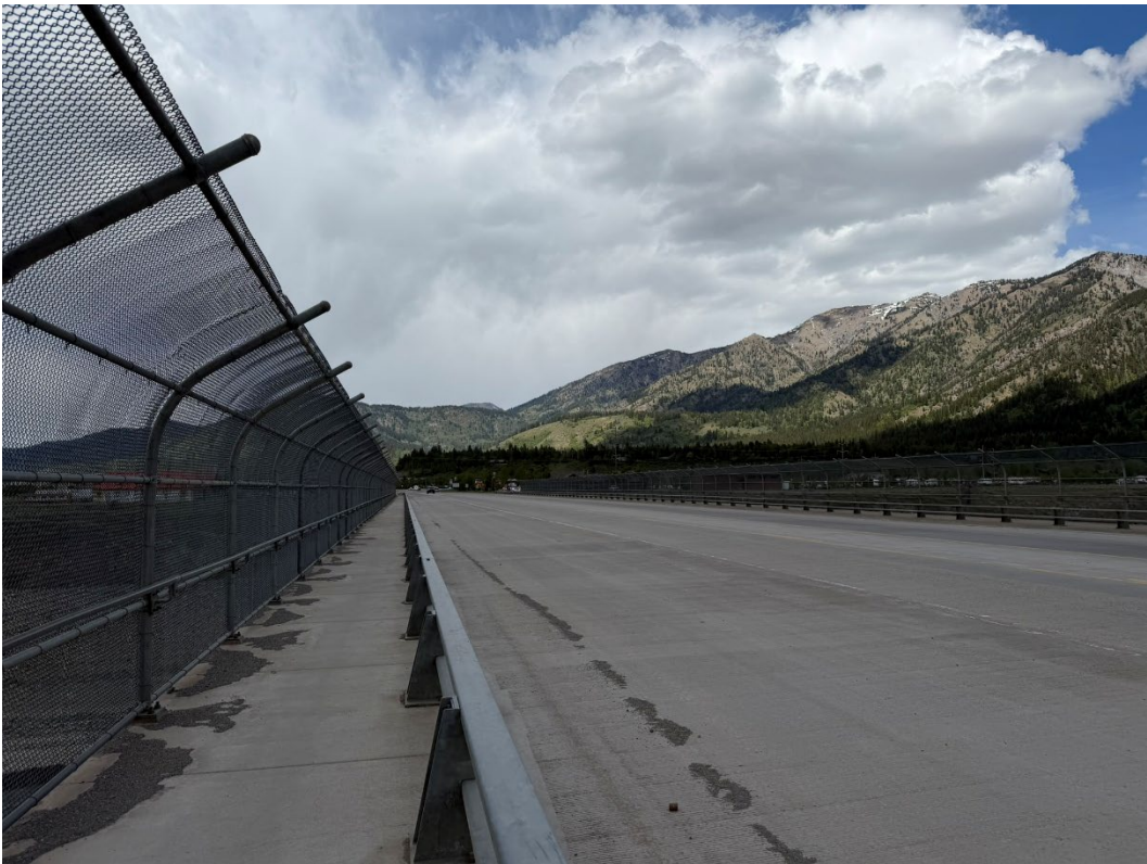
Figure 7. US 89 Bridge Crossing Snake River
