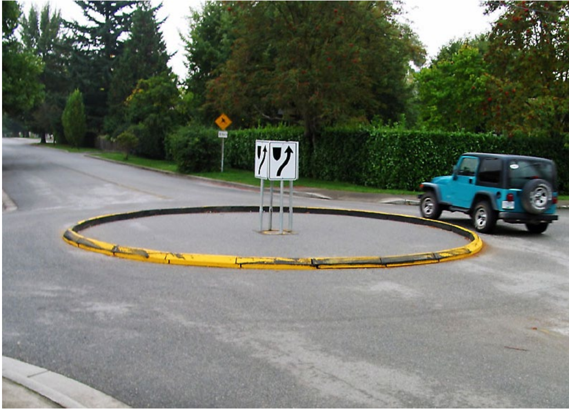
Figure 18. Example of a Temporary Roundabout Design
